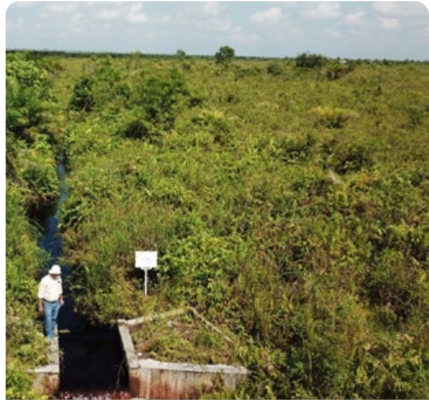
Canal blocking at Jati Mulyo Village area, Jambi
